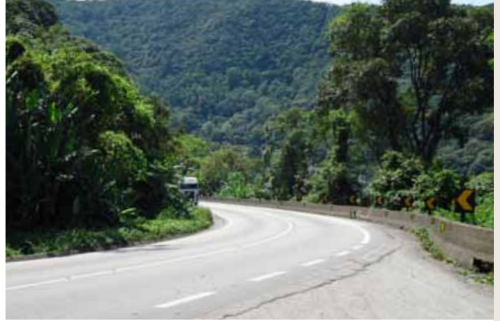
Anchieta Highway, km 44 - km 48, DEGAROUTE® Cold Plastic Structure Marking
