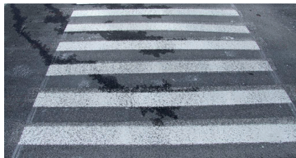
Even after 5 years on the road, the DEGAROUTE® based markings still fulfill the requirements of a Type 2 marking.
