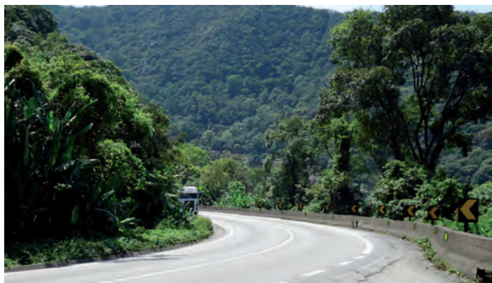
Anchieta Highway, km 44 - km 48, DEGAROUTE® Cold Plastic Structure Marking
