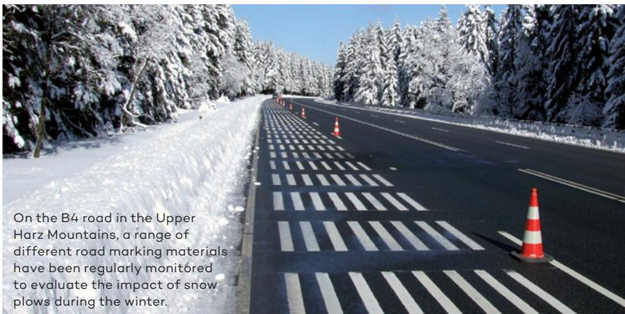
On the B4 road in the Upper Harz Mountains, a range of different road marking materials have been regularly monitored to evaluate the impact of snow plows during the winter.
