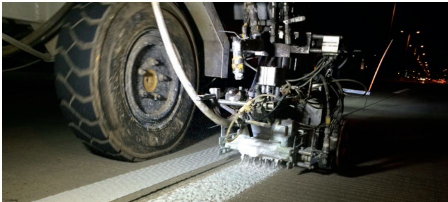
Utilizing specialized equipment, DEGAROUTE® based spray and structured skip markings were applied to a 2-mile stretch of the Illinois Tollway.
