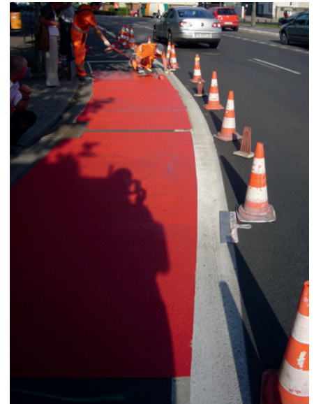
Durable area marking with tailor-made antiskid properties based on DEGAROUTE.
