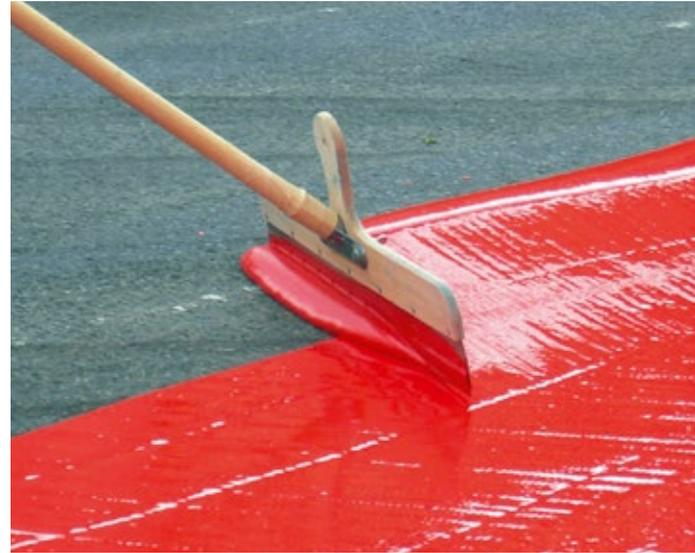
Manual application of a crosswalk, based on DEGAROUTE® reactive resins
