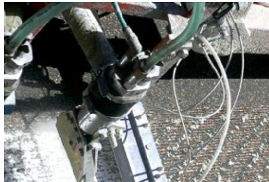
Cold plastics are reactive two- or multi-component systems formulated with DEGAROUTE® binders based on methyl methacrylate (MMA) and brought to polymerization by the addition of the curing component (hardener) immediately before application. The system cures chemically after a certain lapse of time (pot life), when the volatile resin components are chemically bound in the resulting inert duroplastic polymer. Thus application can be considered to be almost **free from VOC emission**.
